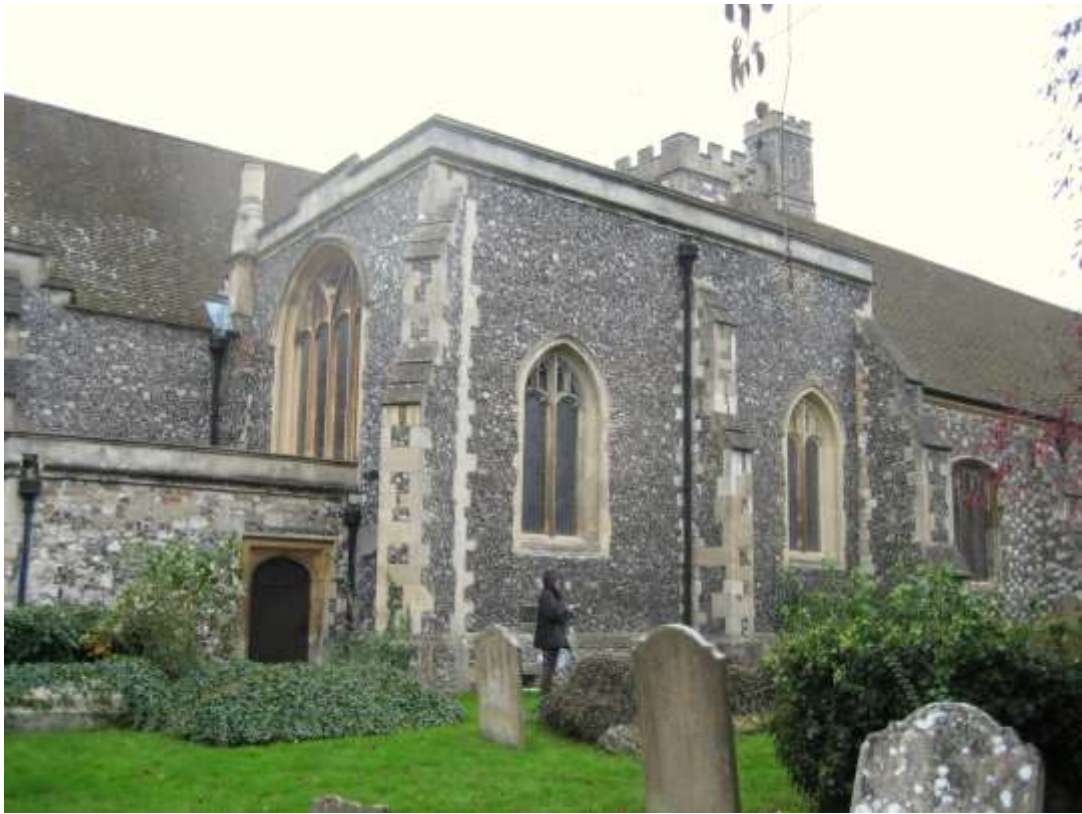
The Norreys Chapel at the east end of the north aisle of St Michael's Bray
