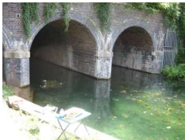
Site 4 At the Railway Bridge (photo 12/7/20)
