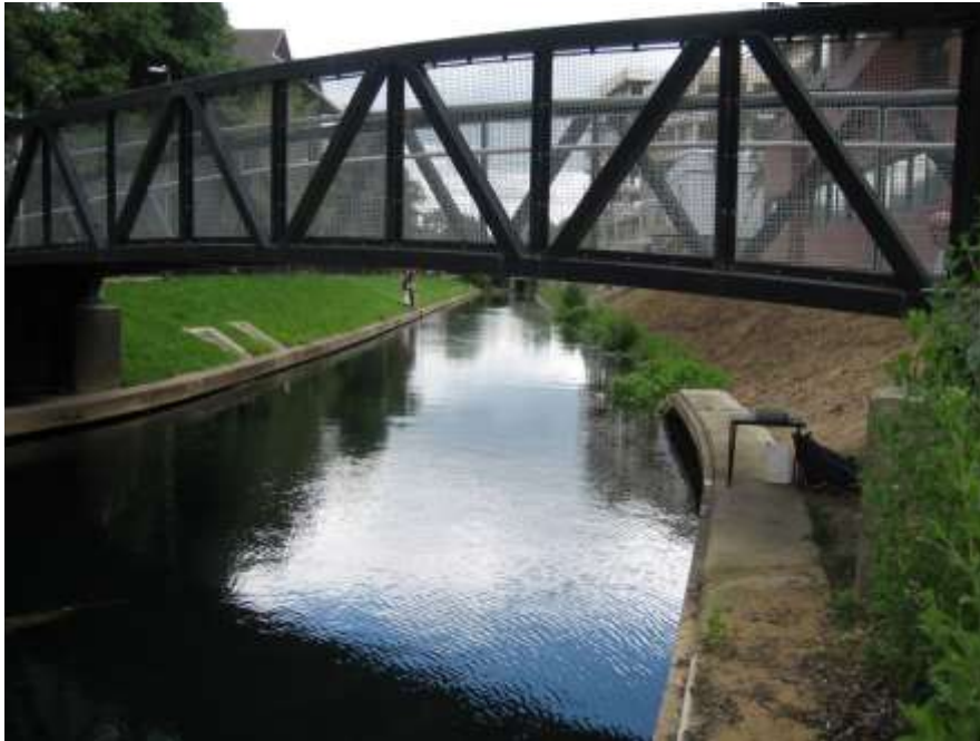
Site 2 At the Library Bridge (photo 19/6/20)
