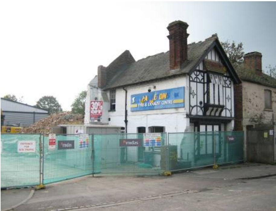
Demolition at the former Stapleton’s site in Moorbridge Road now underway
