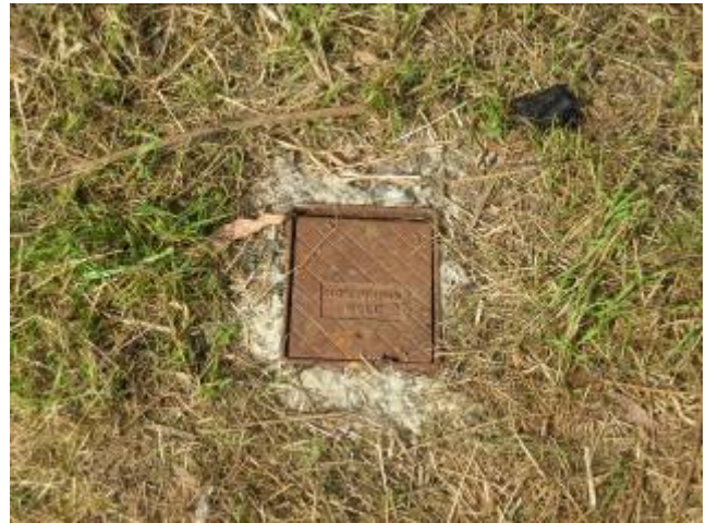
Monitoring well cover plate uncovered by weed clearance
