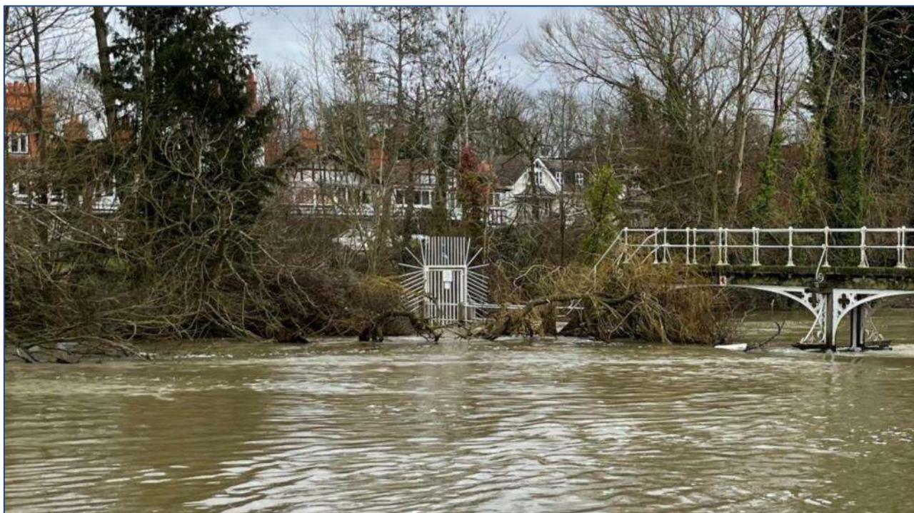
The river in full flood in mid-February, clearly showing the build-up of damaging debris abutting the island end of the bridge
