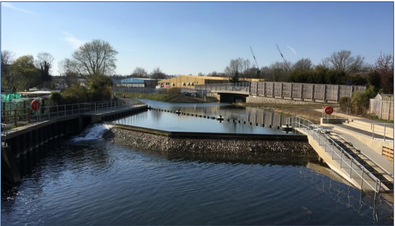
The newly opened weir at Green Lane
