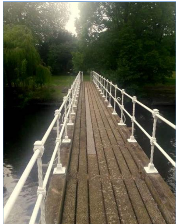
Bright new railings now adorn the bridge
