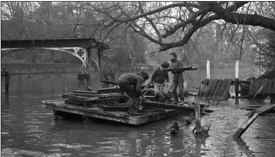
Volunteers clear away rotten timbers from the bridge deck near the island
