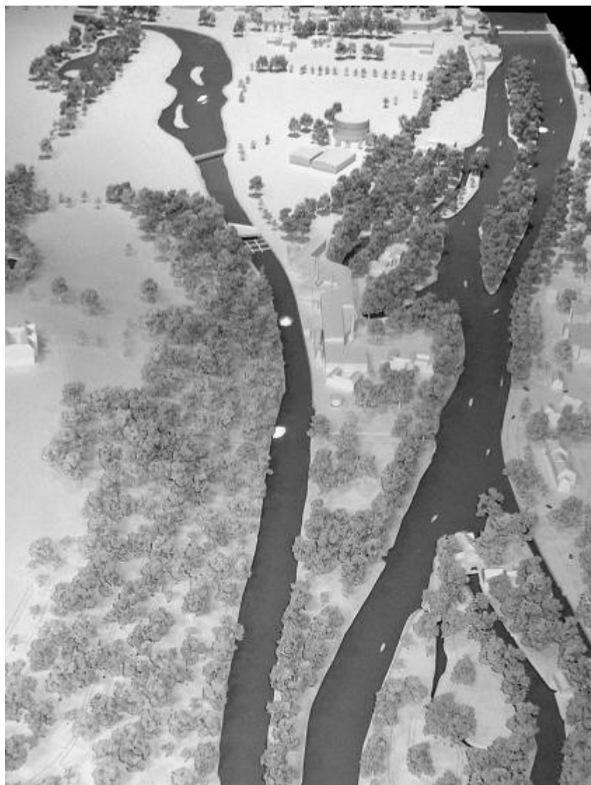
The 48-acre site occupies most of the land between the two waterways. Looking south, with Maidenhead Bridge in the top right corner.
