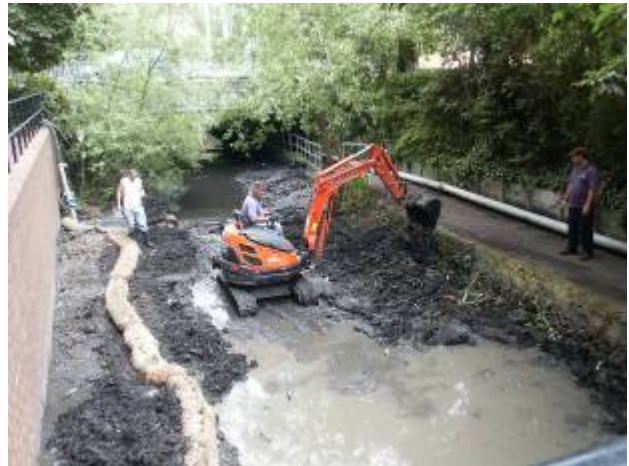
1 st June: digging out the channel
