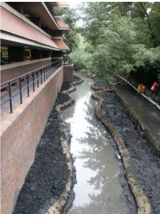
4 th June: meandering stream formed by planted coir
