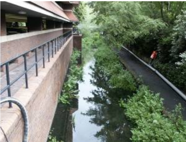
17 th May: York Stream before work started
