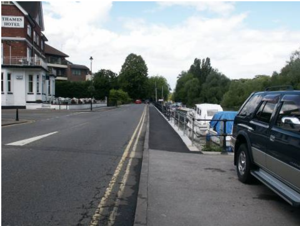
The new pathway opposite the Thames Hotel
