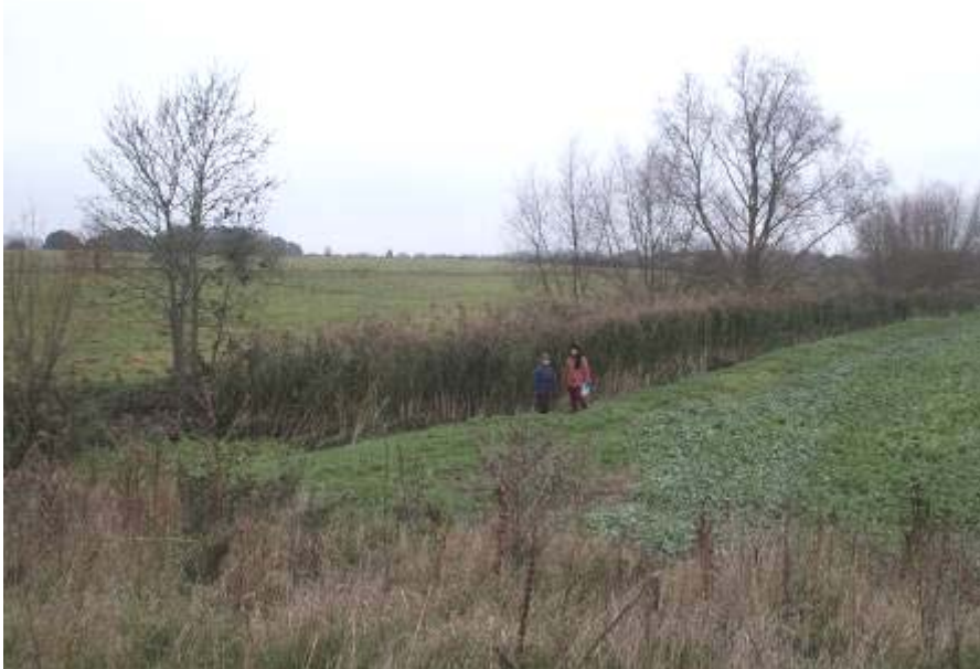
Reeds clogging Maidenhead Ditch, north of the flood control gate, November 2005
