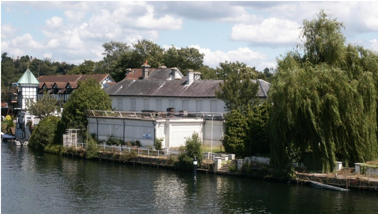
The progressively deteriorating Skindles Hotel site, which recently suffered further ignominy when the chimney collapsed.
