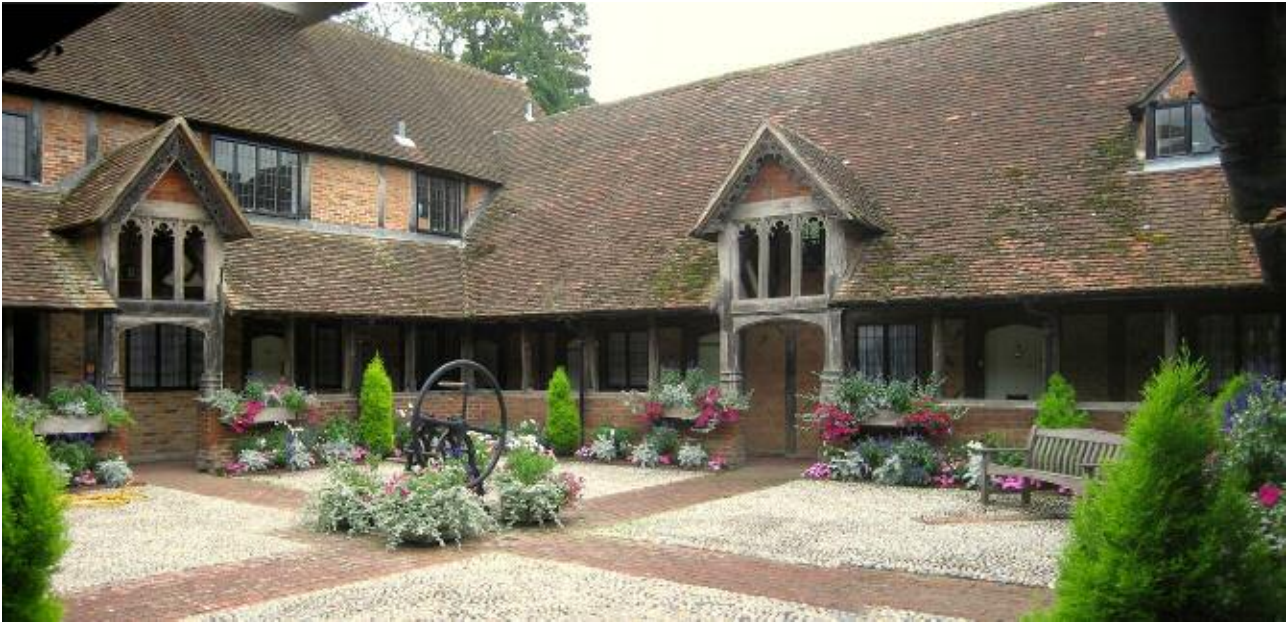
Ewelme Almshouse founded 1437, built by 1448. The bargeboards on the porches are very similar to those of Ockwells Manor build ca. 1450
