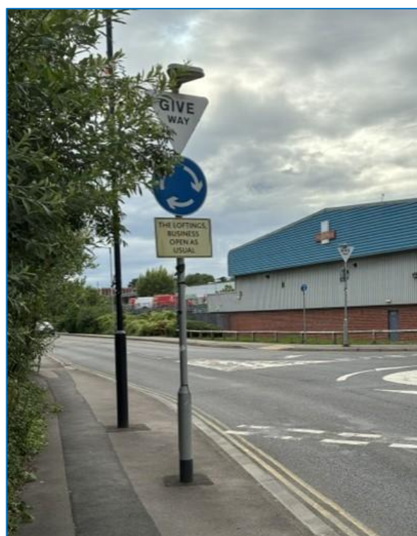
The Loftings were completed in 2019. The red border on the “give way” sign has completely faded. The give way sign on the opposite side of the road faces the wrong direction and has been in this state for over a year! This is on the busy Stafferton Link road.
