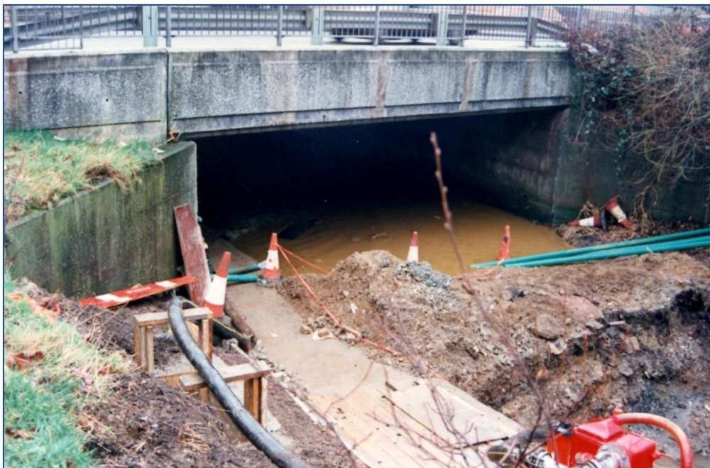
Ditch being dug for cable in the stream bed in 1992
