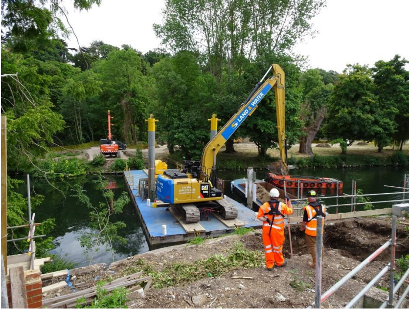
Excavations prior to installing the footings of the bridge on the island
