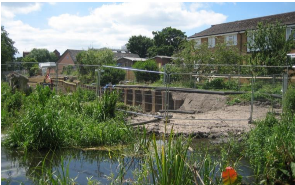
Earth dam on Town Moor, presumably added to the earlier barrier, (see Newsletter Aug 2015) to prevent water flow into section north of A4 now being worked on
