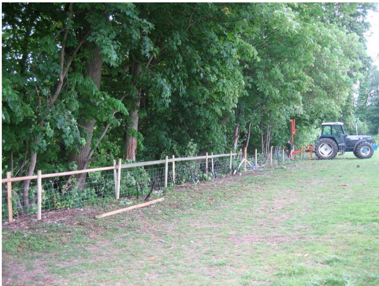
Putting in the fence at the edge of the chalk pit
