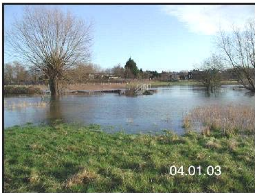
Flooding next to the nursery in 2003 after the flood bund was constructed (Photo courtesy Margaret Bowdery, East Berks Ramblers)
